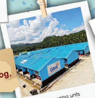
120 housing units For the survivors of Typhoon Sendong
