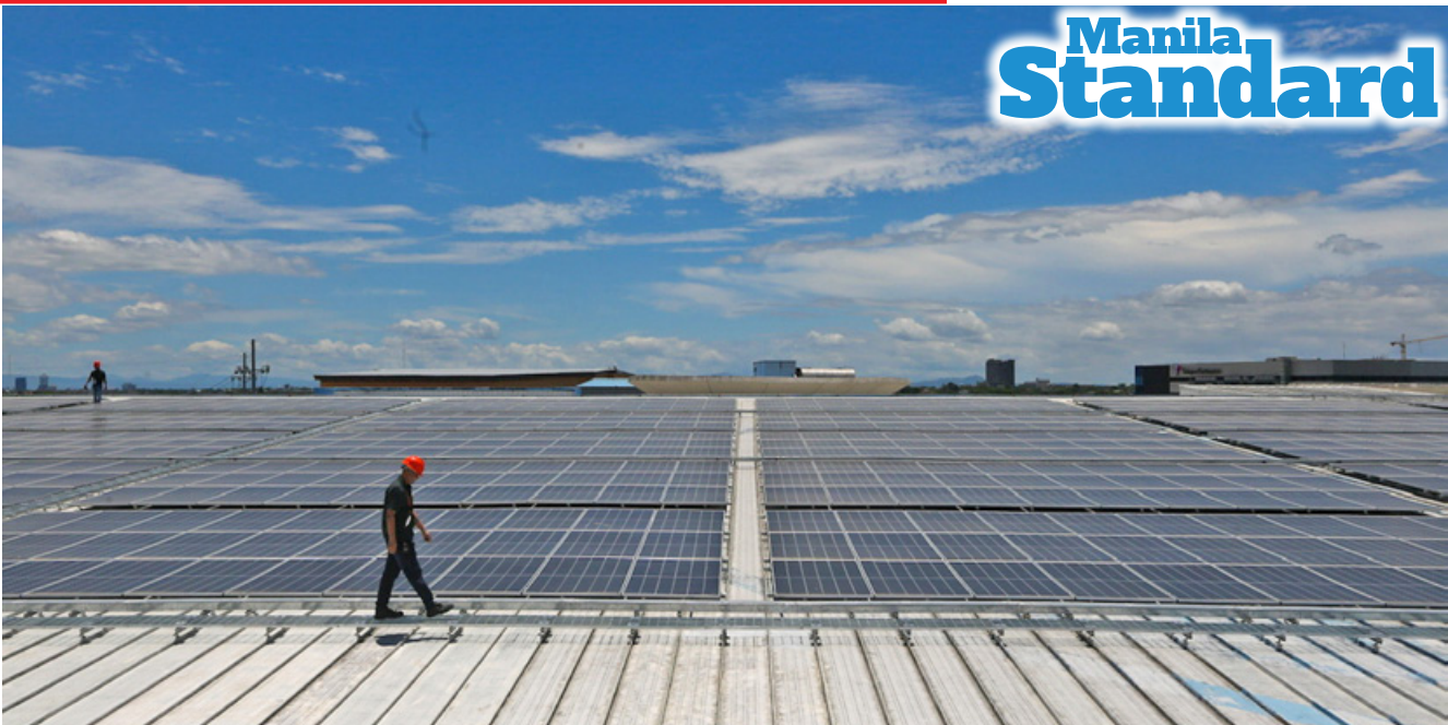
SOLAR ROOFTOP. Workers inspect the 3,638 solar panels installed across the 9,328-square-meter rooftop of SM city Molino on Sunday, April 27, 2025. With a direct current capacity of 2,000.9 kilowattpeak powered by 13 inverters, the solar installation can supply energy equivalent to powering 1,500 to 2,000 residential households. This initiative not only supports environmental conservation but also delivers big savings, helping the mall reduce its annual power bills by up to P12.4 million. Norman Cruz
