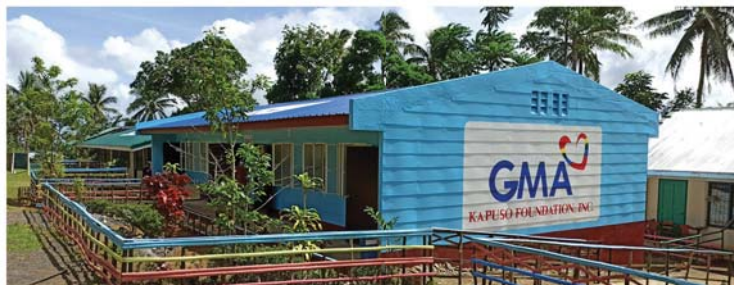
San Rafael Integrated School Brgy. San Rafael, Prieto Diaz, Sorsogon
