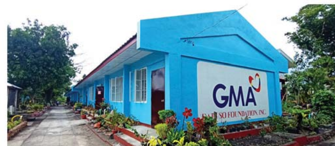
Sto. Domingo Central School Brgy. Sto. Domingo, Virac, Catanduanes
