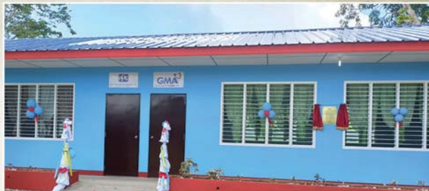
Abariongan Uneg Elementary School Brgy. Abariongan Uneg, Sto. Niño, Cagayan
