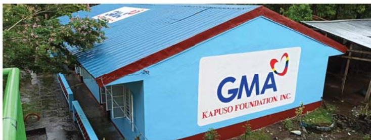
Bariw Elementary School Brgy. Bariw, Camalig, Albay
